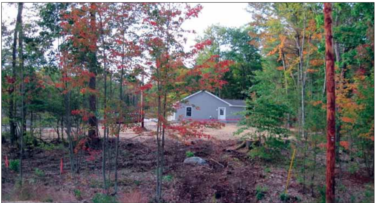
LEA found cases where rain gardens weren't installed and a house (above) was built inside a buffer.
