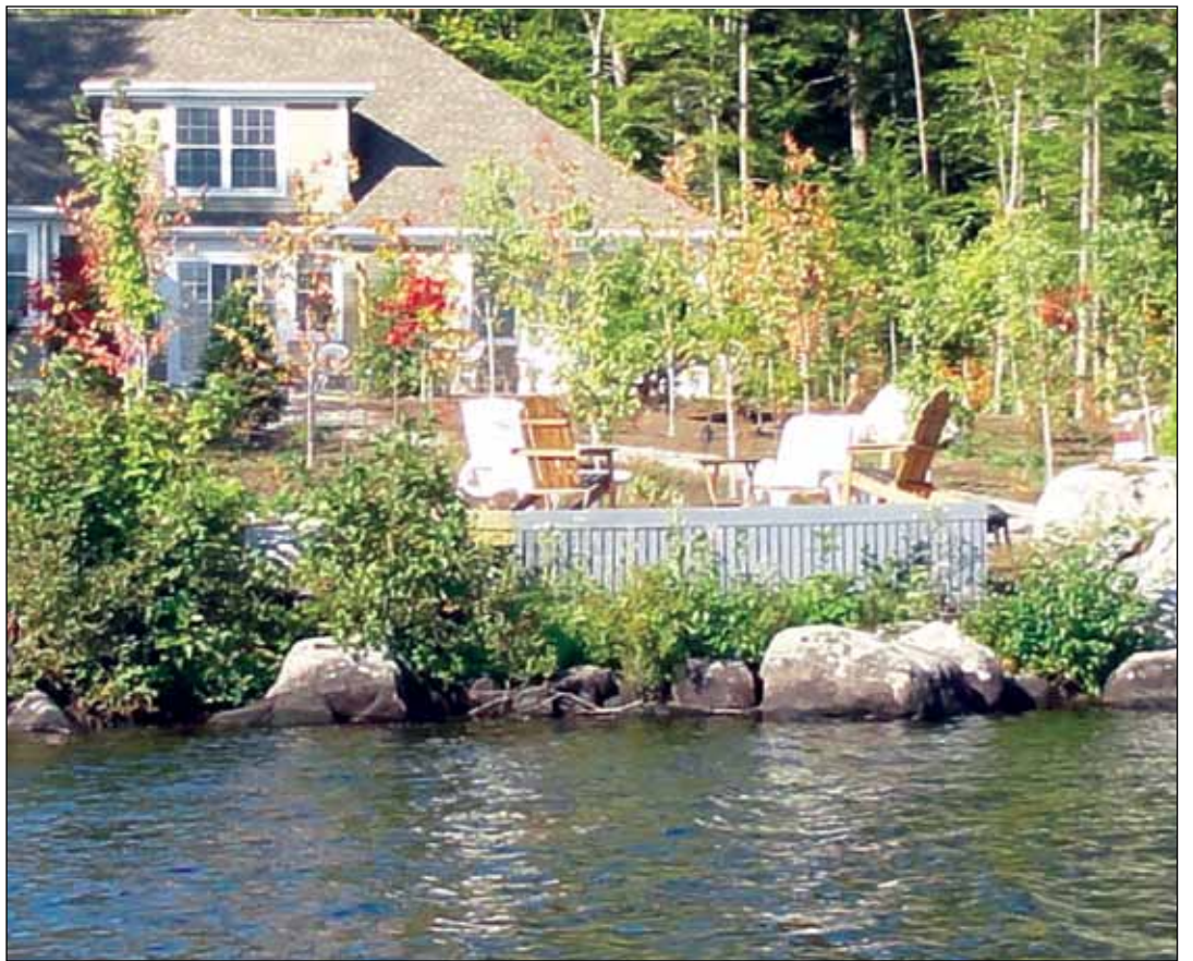
The Chase property on Long Lake before the illegal patio/deck was removed.
