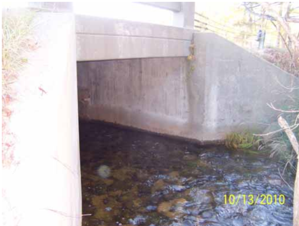
4. Outlet structure (downstream side)
