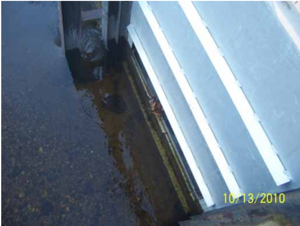
1. West gate of dam
