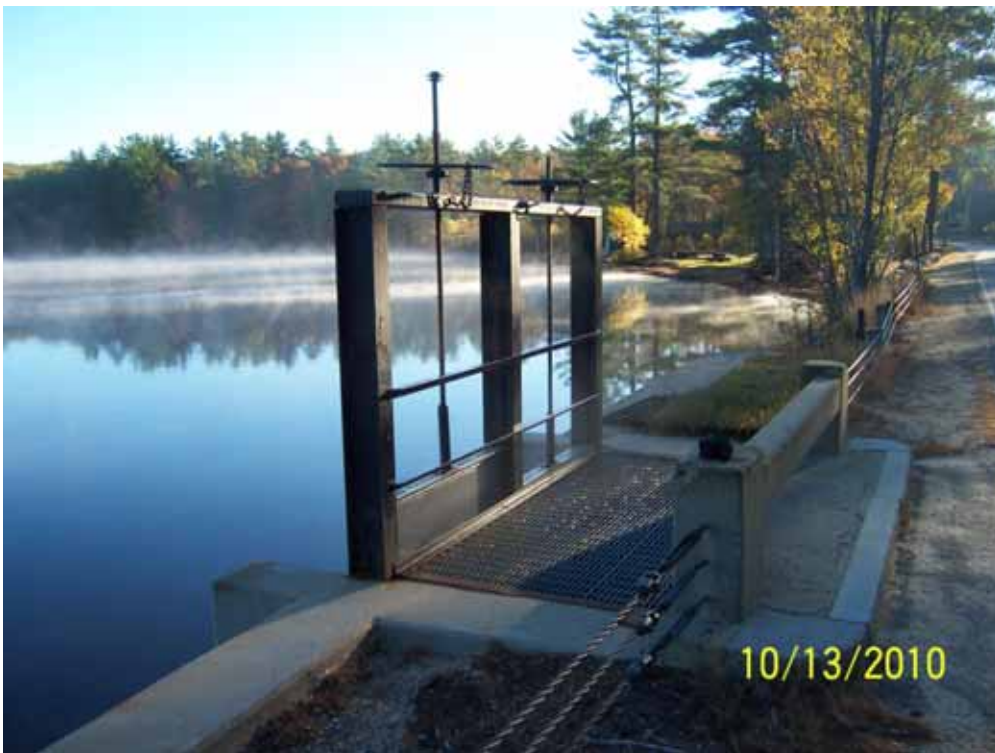
2. Dam from west headwall
