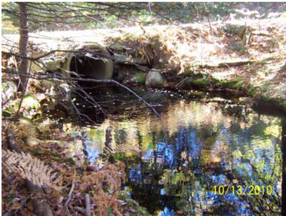
16. Wildwood Road grade (gravel) adjacent to Sucker Brook bank edge
