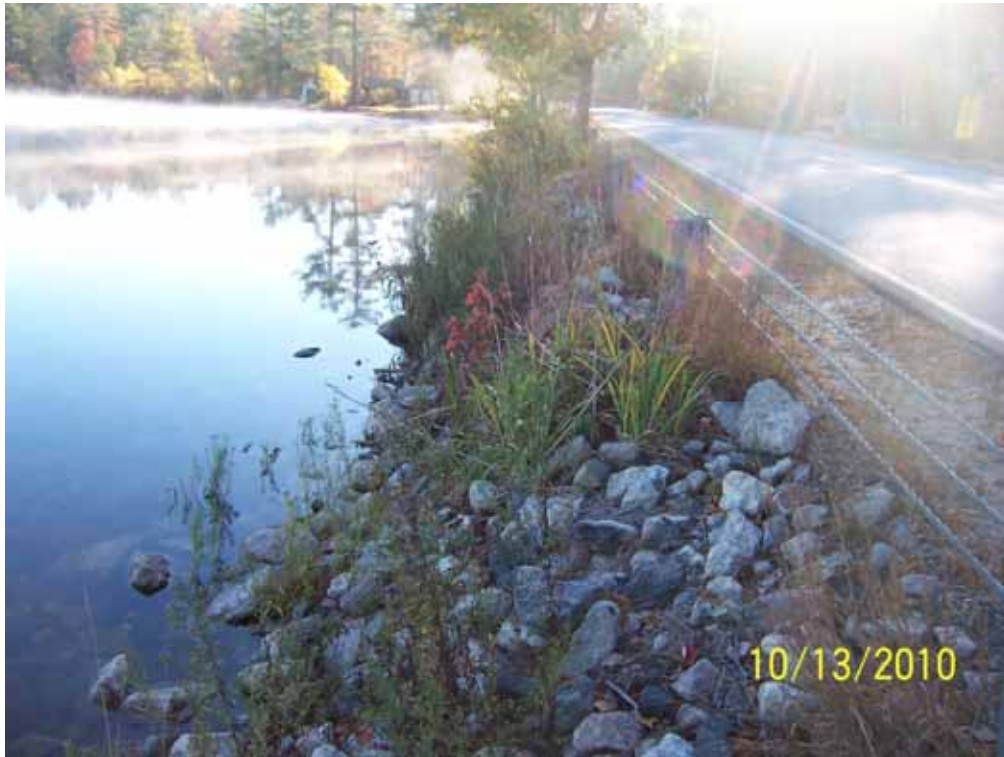
5. Rip-rap at edge of causeway
