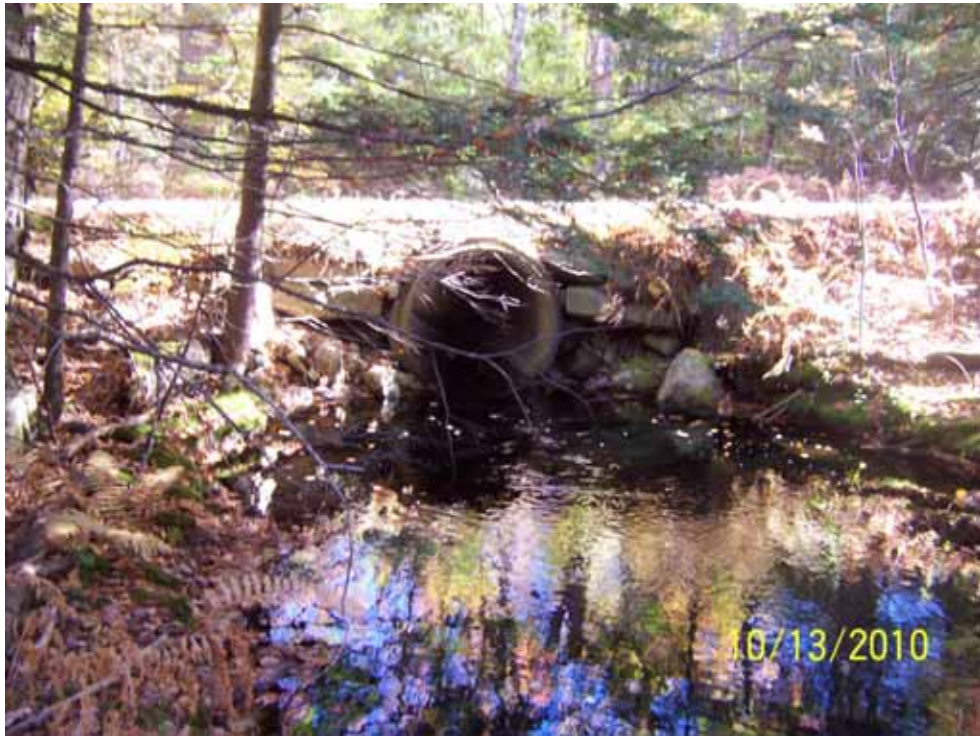
15. 60" dia. Culvert outlet on Sucker Brook under Wildwood Road
