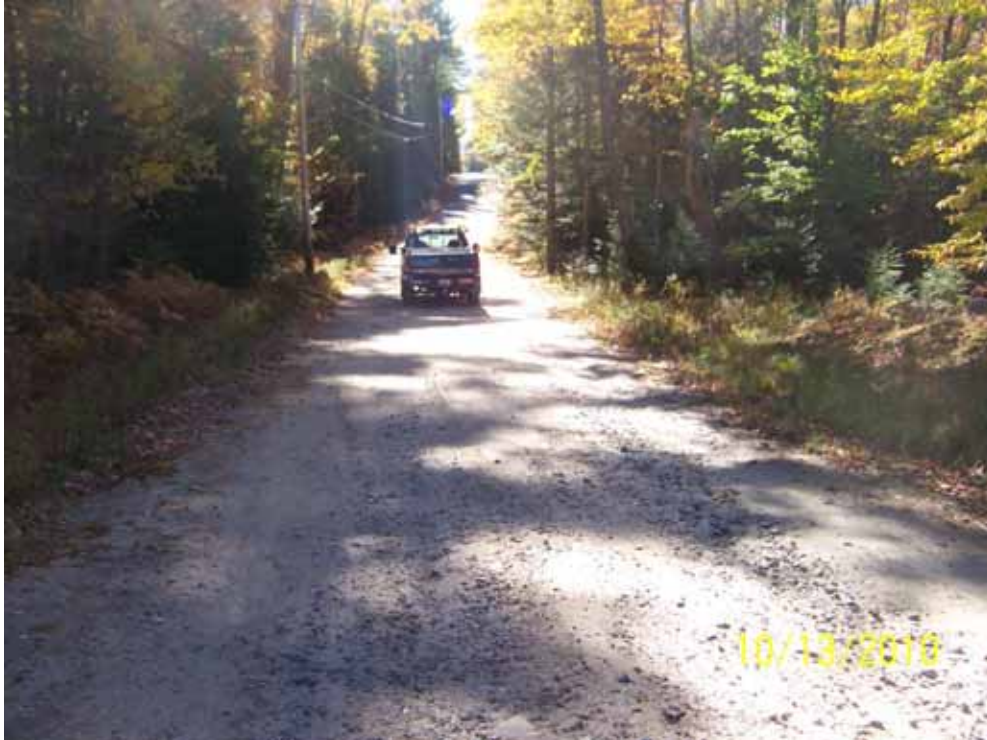
17. View southerly down Wildwood Road (note fine sediments accumulated and migrating off right side of road)
