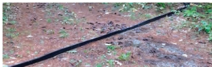
Driveway With Razor Installed
